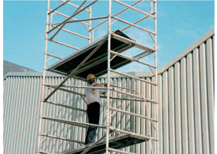
Wall cladding being over-painted.
